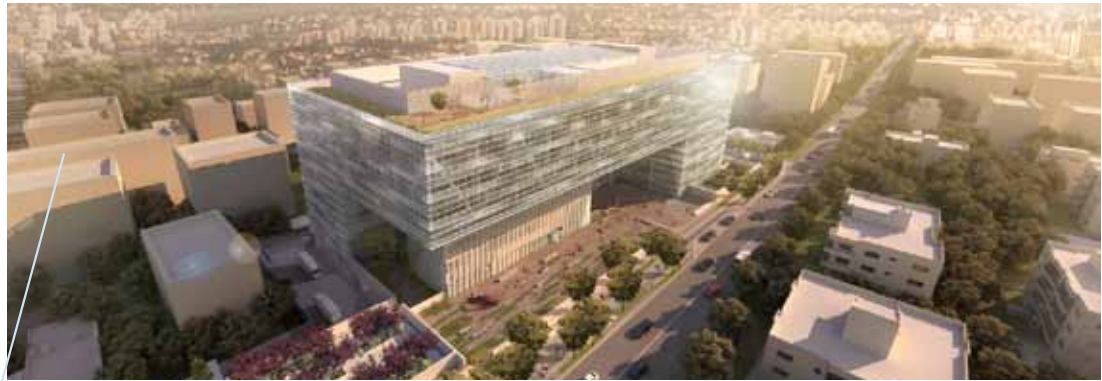
External 3D Shot - New Headquarter Building Project "Shemeisani"
