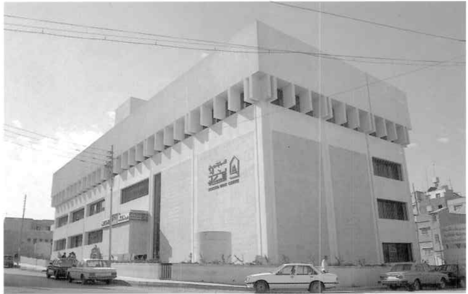
The Housing Bank Centre in Zarqa
