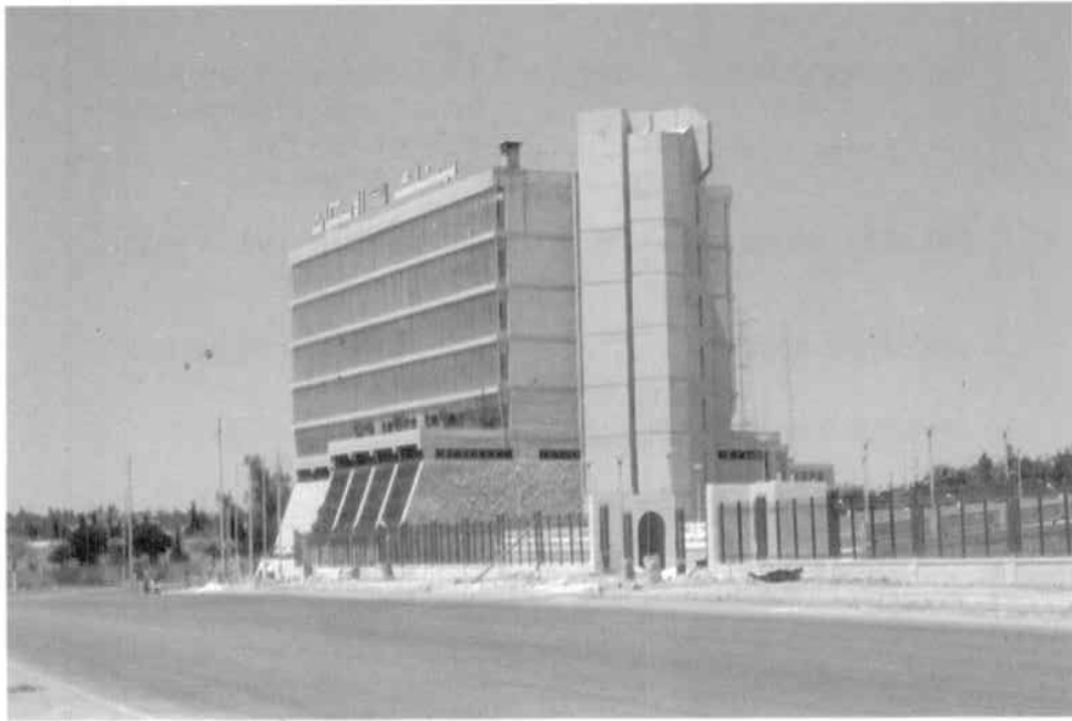
Bank Headquarters in Amman
