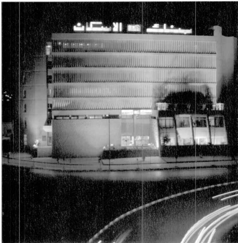
Bank's Headquarters in Amman
