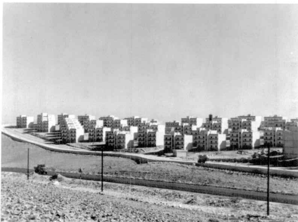
A Housing Scheme for low Income constructed by the Housing Corporation And Partially Financed by the Housing Bank
