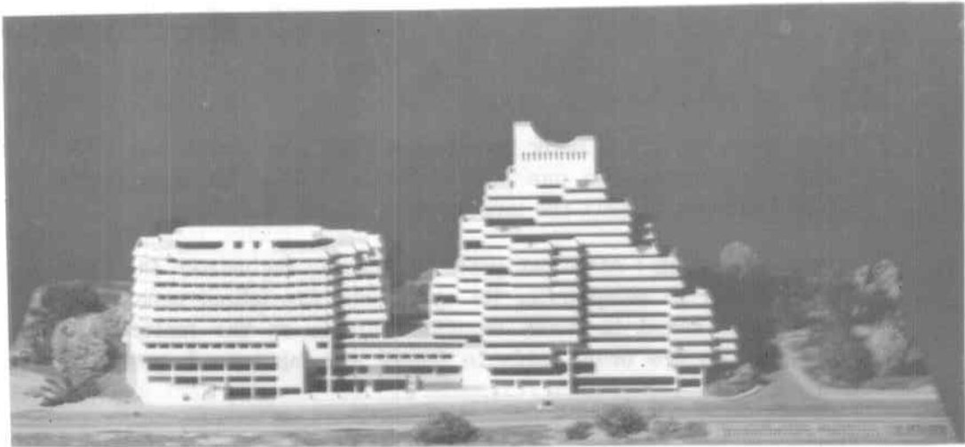
Commercial Centre Project - Shmeisani - Amman Under Construction
